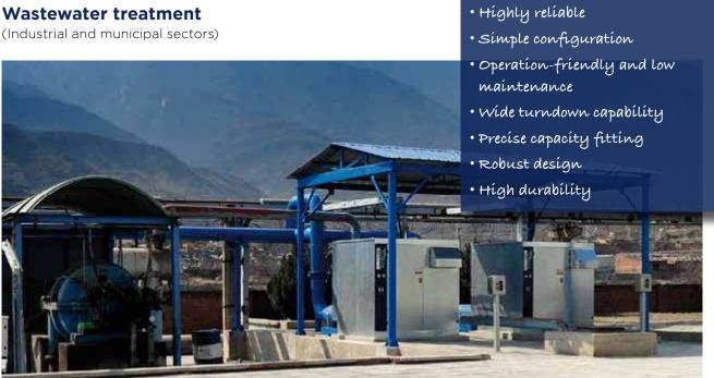
Modern wastewater treatment requires the movement of large volumes of air at low pressure and Robuschi's PD blower range provides a reliable source of air for its different processes.
