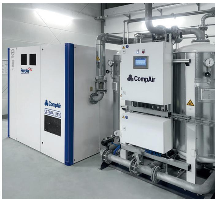
As part of the subsequent performance qualification process, the team then collected data over the course of a month to ensure that the compressed air remained impeccably clean. In the meantime, the compressed air system is up and running, and dew point or oil-free levels are continuously recorded online, while discrete measurements on particles or bacterial counts are taken at regular intervals.
