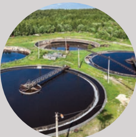
Sewage Treatment Plant for aeration
