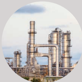
Chemical Factory for air transfer
