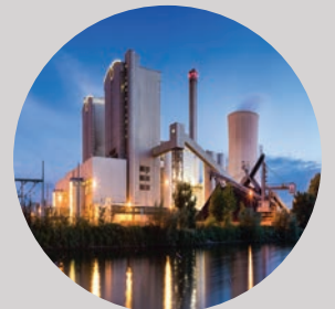
Power Plant for supply oxygen
