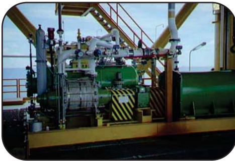
NASH 2BG Compressor used for vent gas compression on an offshore rig
