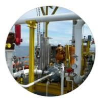
An FGR system is designed to capture waste gases that would go to the flare tip during normal operations. The FGR system is located upstream of the flare to capture and recover some or all of the waste gases before they are flared. Most flares operate at pressures just above atmospheric pressure, and therefore the gas must be compressed to a higher pressure for transport throughout the plant and for use at the intended destination.
