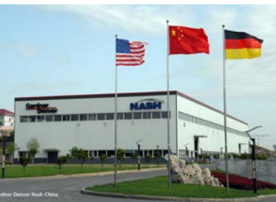
The Gardner Denver facility in Boshan, China, manufactures liquid ring vacuum pumps and multistage centrifugal fans for a global customer base.
